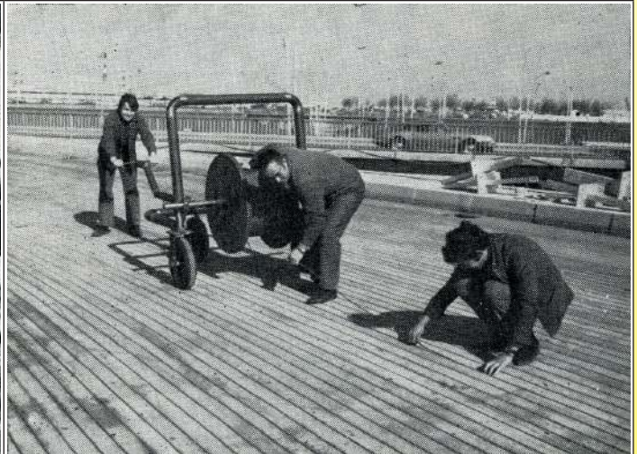
1968 Installation of the heating web on an access ramp to a bus parking platform, Orly airport near Paris (Electric floor heating, by Robert Félix, 1971, Ultimheat Museum*)
